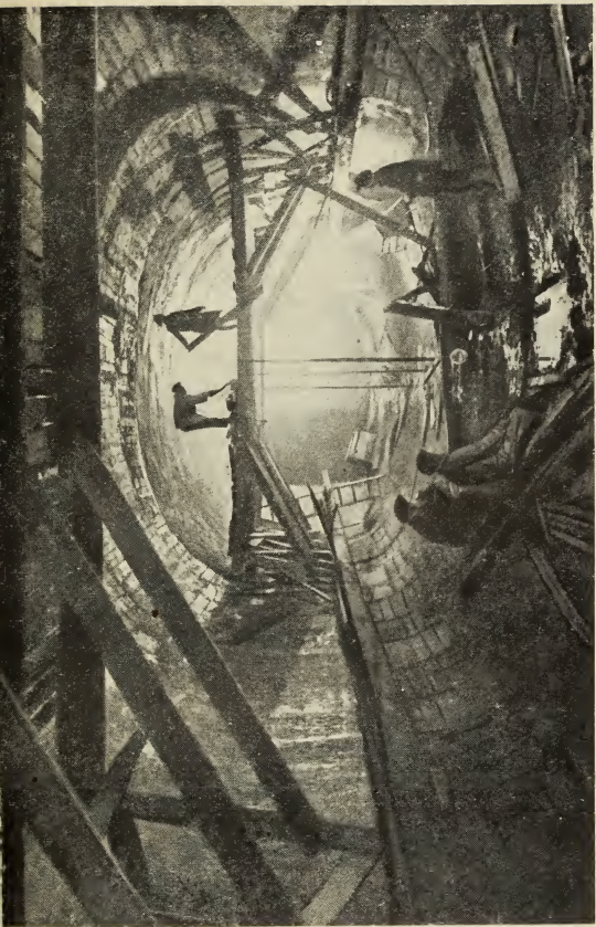
The Finishing Work in the Tunnel
